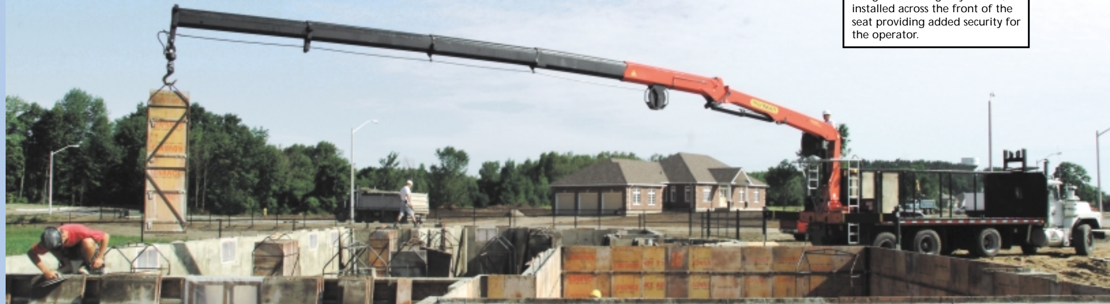
PowerLink™ linkage system gives the outer boom added strength in flat-out position and a constant folding speed.
