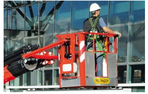
PERSONAL PROTECTION AT THE BASKET ENSURES SAFE WORKING
